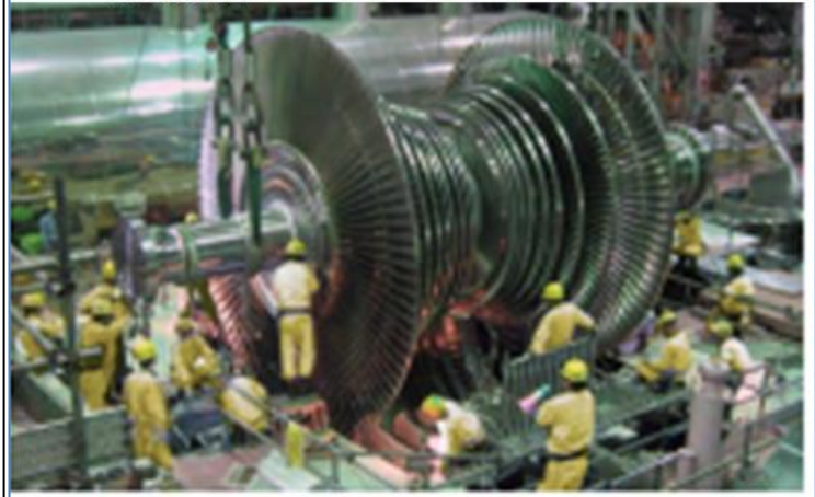
Turbine Installation
